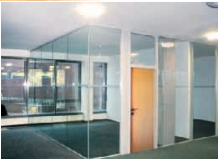
All-glass wall with door and transfer port element for ventilation
