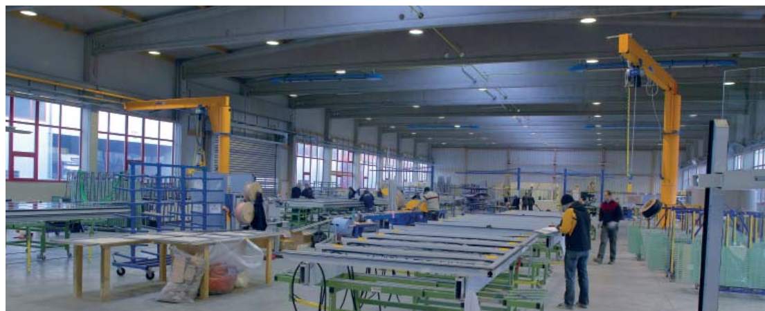
Final assembly of facade elements
