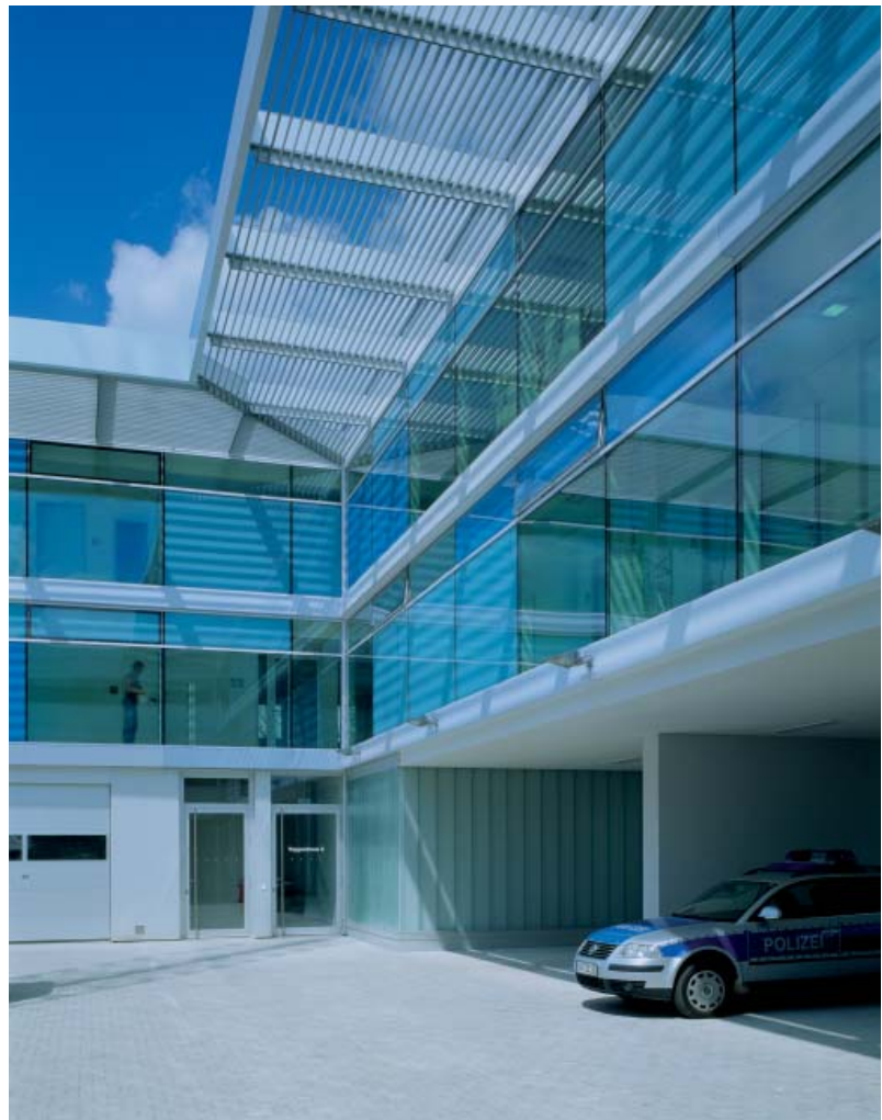
Police station, Barnim
